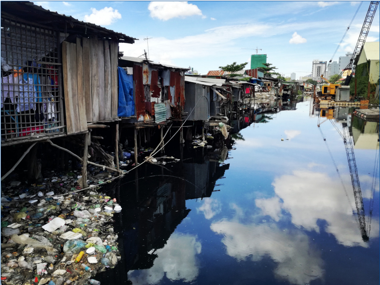
Figure 3 Part of the sewer making its way along the road and the sign shown above. Source: Author.
